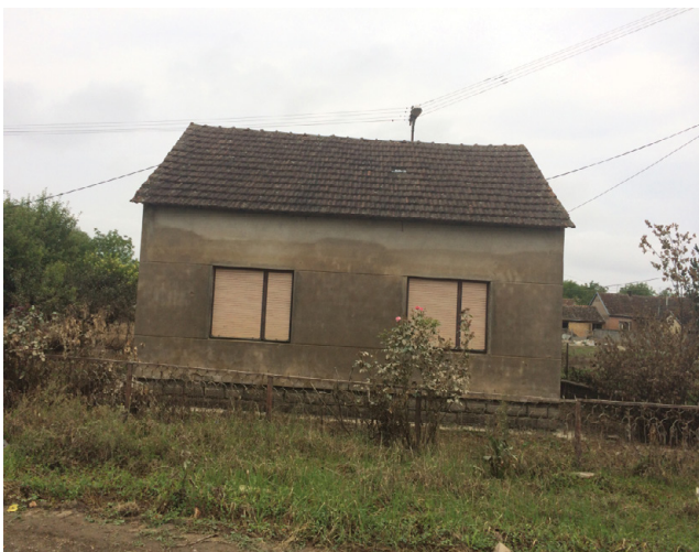
Figure 5: Water level in flooded area Rajevo selo.
