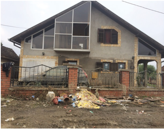
Figure 4: Flood affected house in village Gunja.
