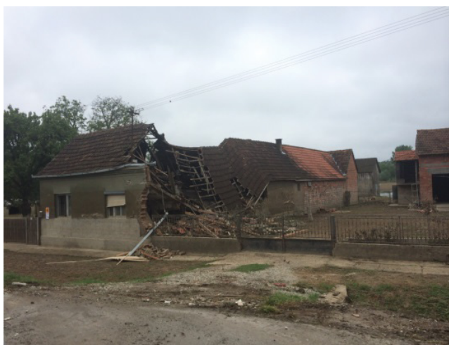
Figure 6: The damage magnitude in village Račinovci.
