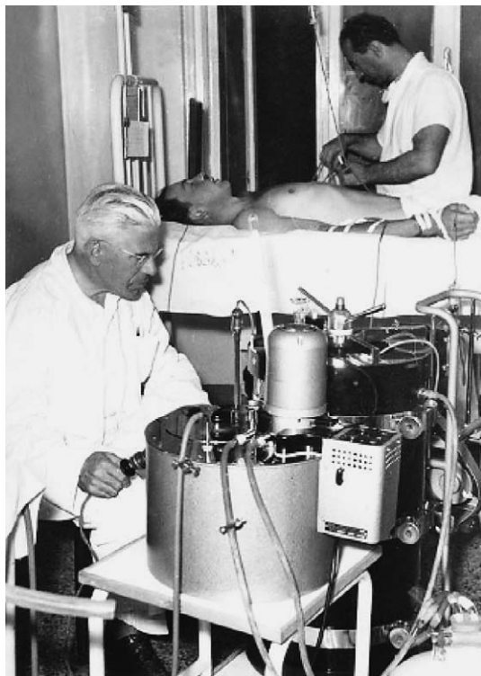
Fig. 1. First hemodialysis in Slovenia (1959) with Prof. Rakovec next to the dialysis machine.
