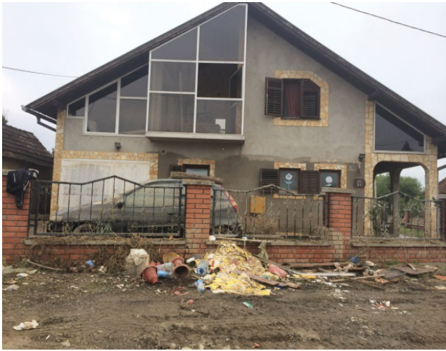
Figure 4: Flood affected house in village Gunja.
