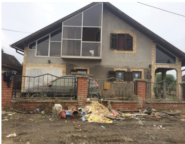
Figure 4: Flood affected house in village Gunja.
