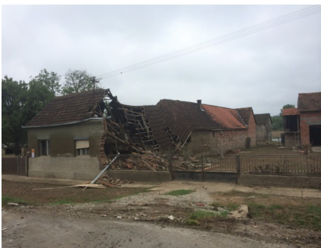
Figure 6: The damage magnitude in village Račinovci.
